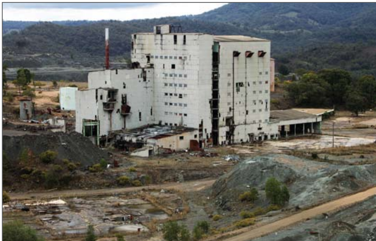
Photo 1. Abandoned mill house.
